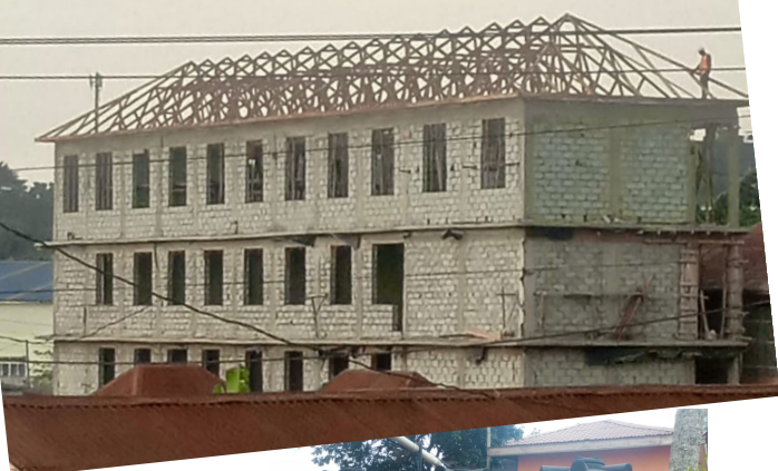
Above: the new school building
